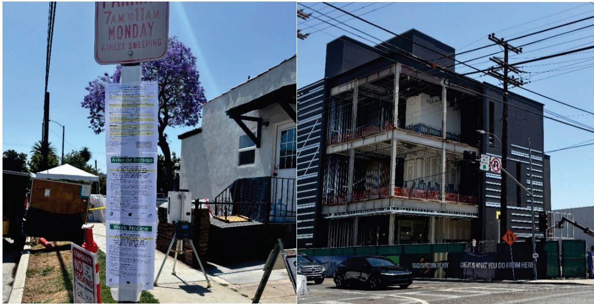
Figure 2: From left to right, home undergoing soil remediation from lead exposure; Data center under construction in close proximity to sterigenics facility in Vernon.
