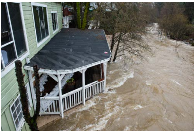
Flooding from Deer Creek reached Lefty's Grill in Nevada City during the atmospheric river storm on January 10, 2017.
