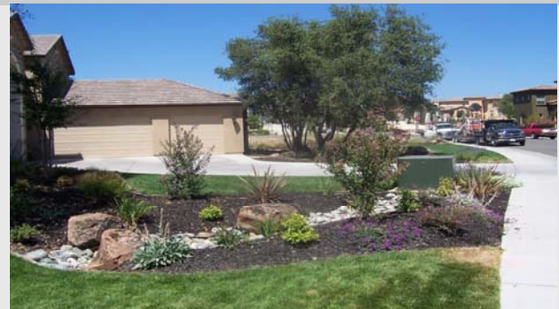
Rain Gardens and grass swales between houses are used at Douglas Ranch, Granite Bay, CA to catch and filter runoff from roofs and driveways before entering a local stream.
