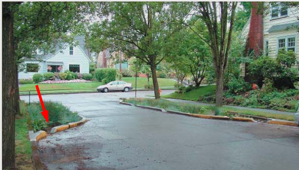
Curb Cuts permit stormwater to flow into grassy swales to reduce roadway contaminants that flow into nearby waterways. They can also be used in existing landscaped areas.
