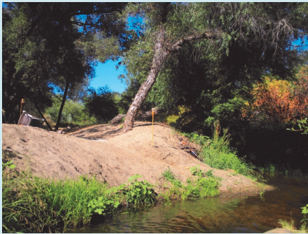
Figure 3. Removal of bank vegetation. Vegetation is often removed by residences to facilitate access. Similar denuding of the banks have been caused by off highway vehicles.
