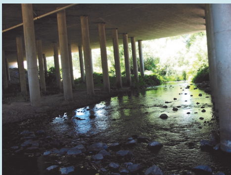
Figure 4. Impervious cover within the creek corridor. Bridges are one of the primary structures that disturb stream corridors. They physically alter the streambed and cause upstream and downstream erosion.
