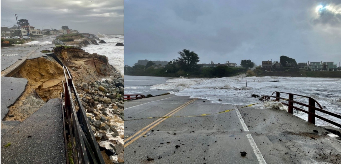
Figure 3.4.4. Storm and flood damage in Santa Cruz in January 2023.
